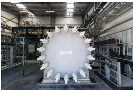
Commissioning of a 2,5MW electrolyser.
